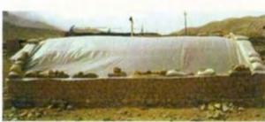
Poly-sheet secured with bags filled with mud, placed on the roof and on the side walls
